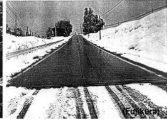
Snow melting: road (heat source: hot water boiler)
