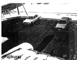
Snow melting: parking lot (heat source: hot water boiler)
