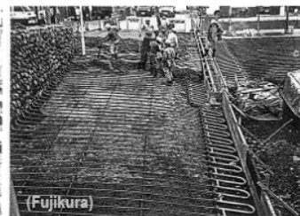
Installation of a road heating system (heat source: hot water boiler)
